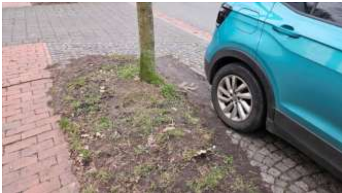
Trees are stressed by conditions with little space and with cars parked on their exposed roots (photo: Glotz-Richter)
